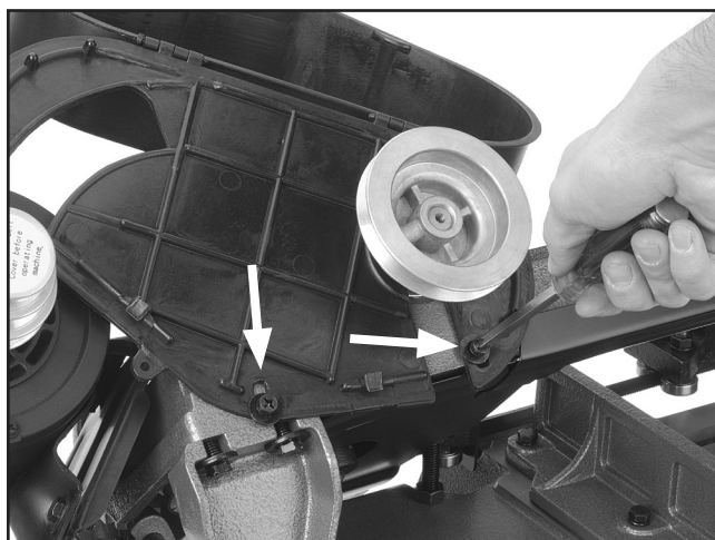
Figure 13. Installing pulley cover.
