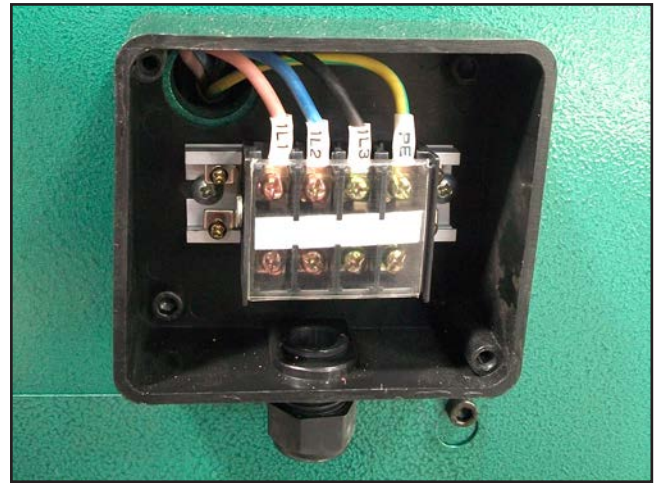
Figure 80. Power-in junction box connections.
